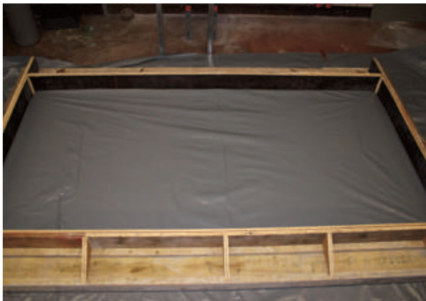
Step 3: Place polyethylene film on top of the elastomer
