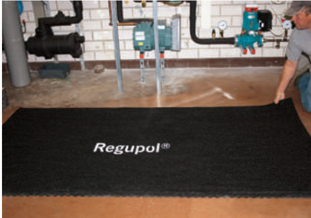
Step 1: Lay out Regupol or Regufoam and cut to size
