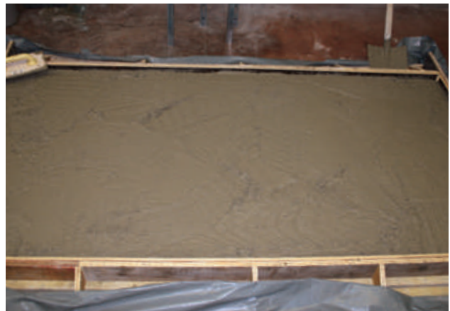
Step 4: Pour concrete into the formwork
